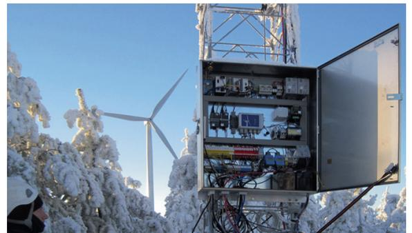
Weather mast for wind farm SCADA systems
