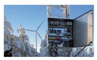
Weather mast for wind farm SCADA systems
